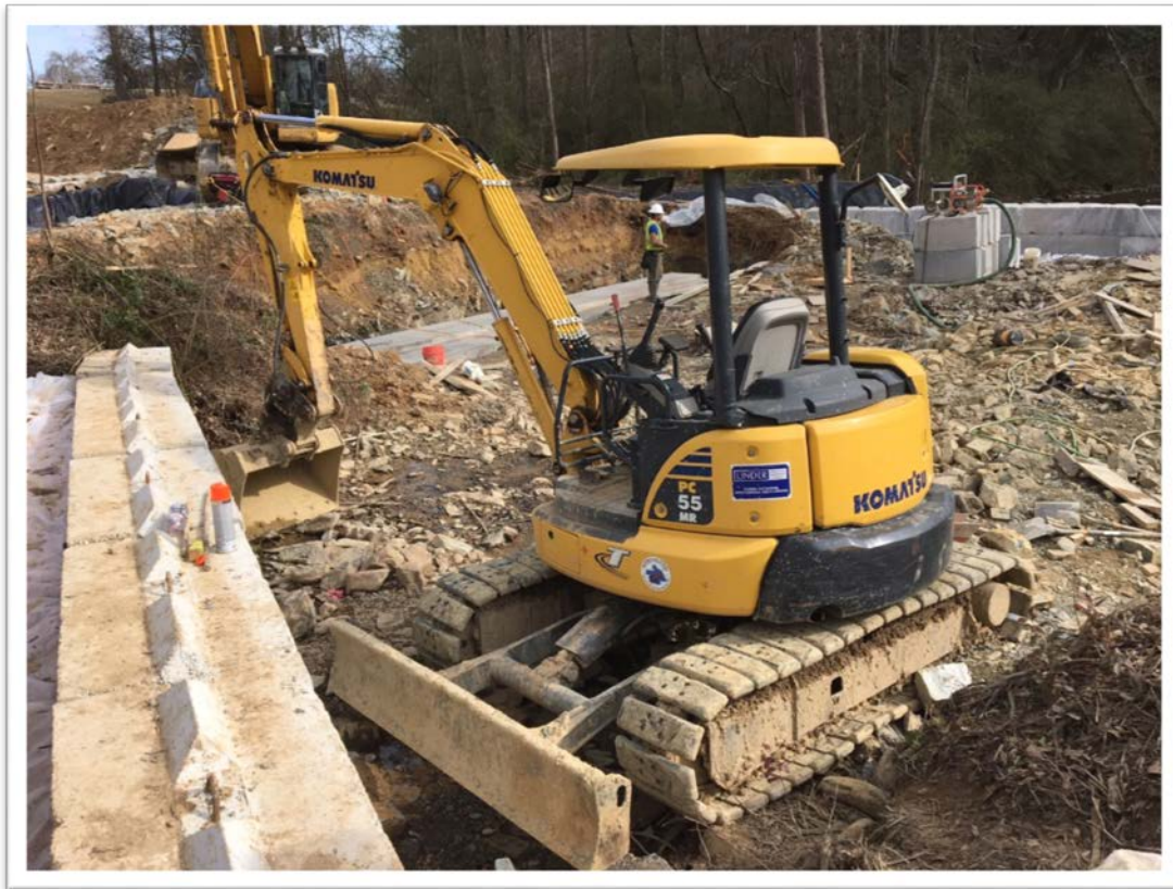
Photo: Lynn Thomas mini excavator replacement funded by GRADE 2013 CMAQ.
